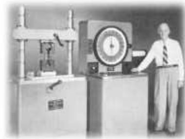
▲ Frank G. Tatnall with later model SR-4 testing machine
