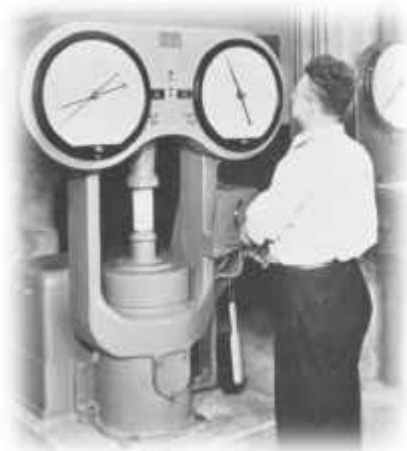
▲ 90,000 lbf Southwark-Emery (compression only) cement testing machine
